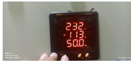
Figure 13 Digital meter showing the dimensions of L2, including voltage, current and frequency.
