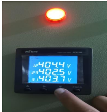
Figure 6 Line voltage of digital power meter (L – L) between R S T or L1 L2 and L3.
